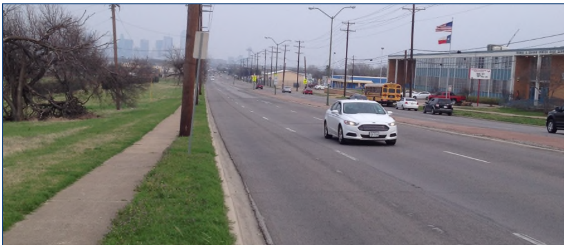
Singleton Boulevard & Project Access - looking east
